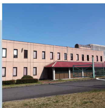
High Fluence Irradiation Facility
